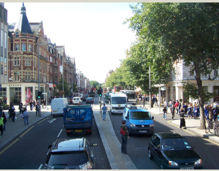
Kensington High Street (two lanes in each direction, variable width median, no dedicated cycle lanes)
